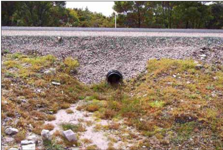
Figure 4: Underpass on the Arthur River Road. (Daryl Polzin)
