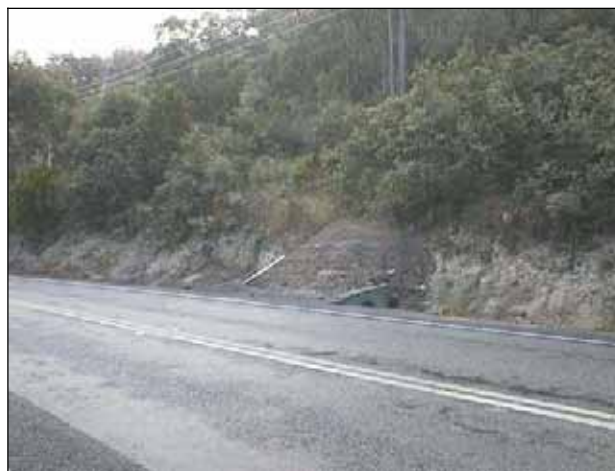
Figure 1: Escape Route Built by DIER on the Arthur Highway. (Taryn Laird)
