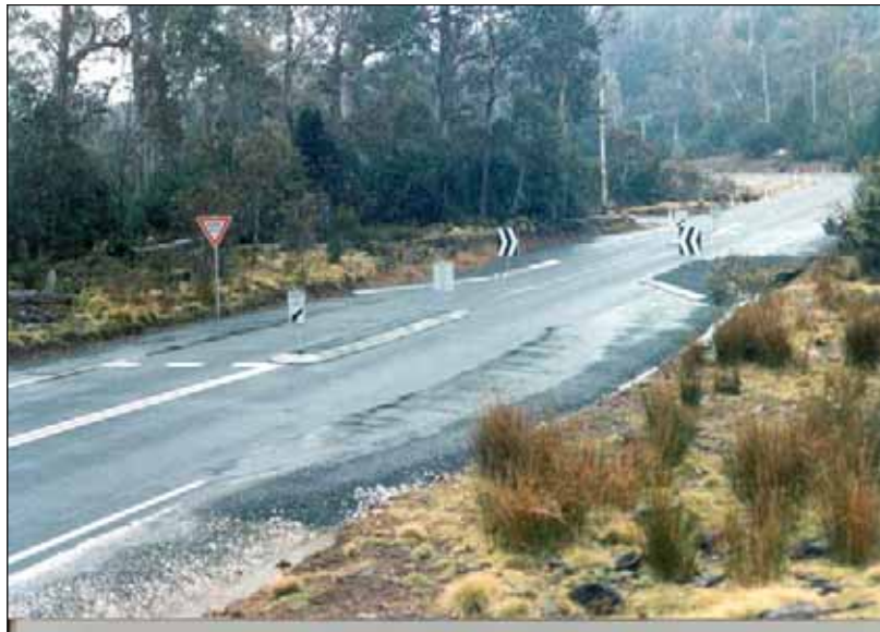
Figure 7: A Chicane Installed by DIER at Cradle Mountain National Park. (Russell Bauer)
